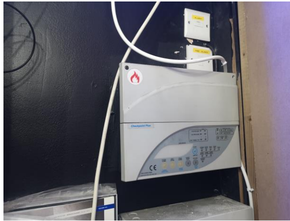
Fire control panel with no power
