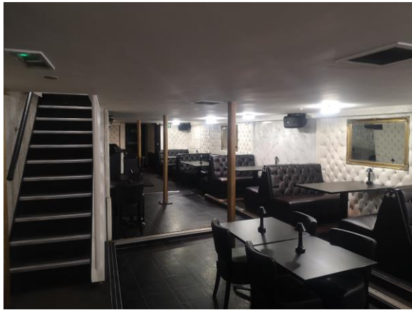
Basement with extensive linings / coverings of an unknown standard
